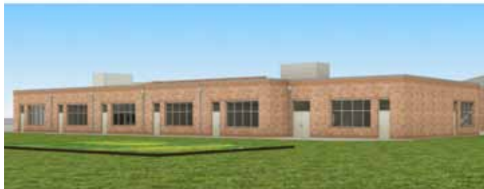
New Meeting Rooms Exterior
