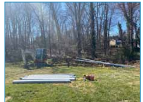
Utility work began in the back of the building
